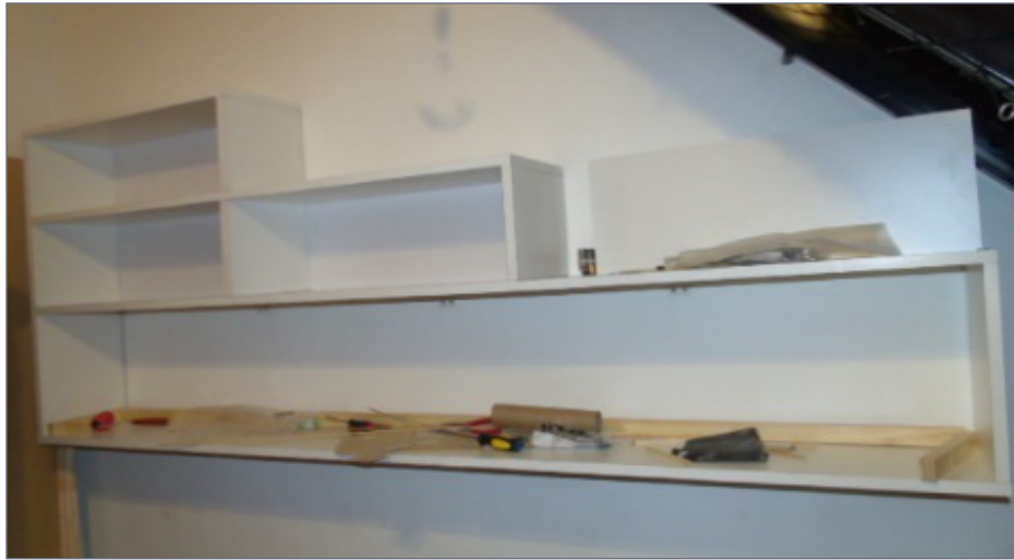
5. The completed shelf structure. It matches the rise of the stairway, and the top shelf is reachable.
